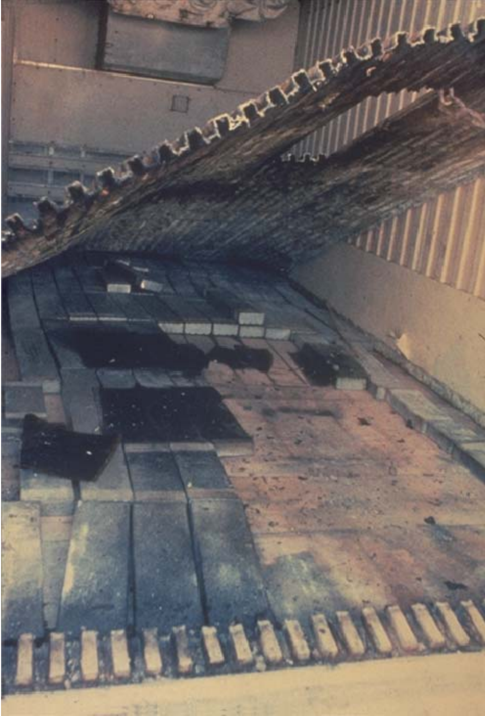
The floor of this refrigerated container was lifted and kilos stacked between the floor and the underside support.
